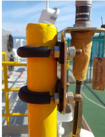
Figure 2: Example of installation to avoid galvanic corrosion.
