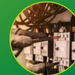
Industrial Electrical Installation and Maintenance
